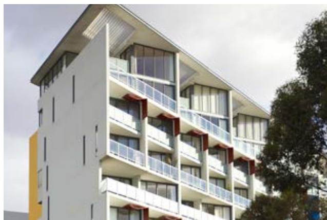
Figure 4Q.7 Natural cross ventilation is facilitated by limited apartment depths and use of dual aspect apartments
