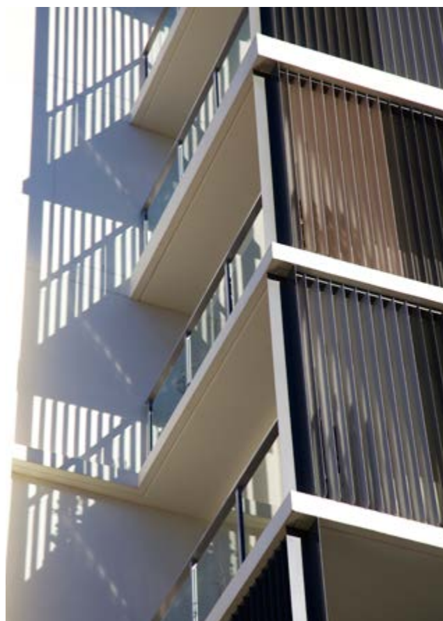
Figure 4L.7 Vertical louvres are an effective sun management technique for east and west-facing windows and balconies
