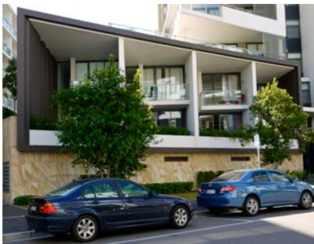
Figure 4P.9 Setting the balustrade back from the building edge allows for landscaping towards the street for increased privacy
