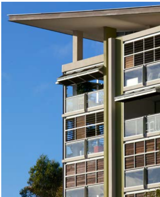
Figure 4Q.3 Operable balcony screens allow occupants to customise their environment and regulate access of natural light and ventilation
