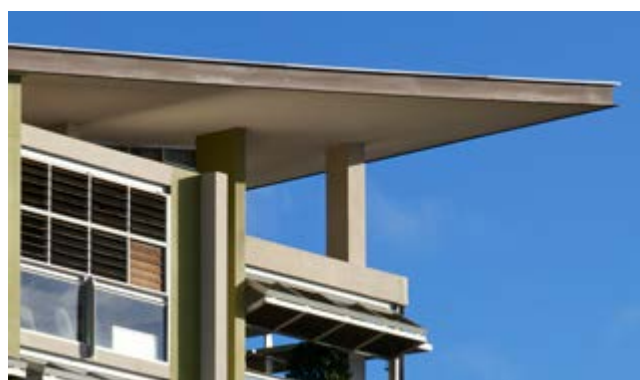
Figure 4D.3 Solar access to apartments can be maximised by tilting roof elements towards north
