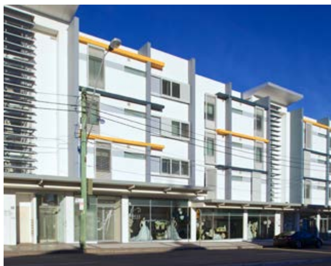
Figure 4T.1 This mixed use development is located on a busy road and is designed with limited openings exposed to the noise source
