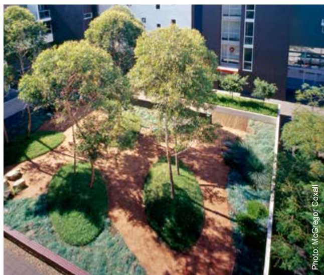
Figure 4F.2 Planting on structures are a way to create open space, in particular where opportunities for deep soil zones are restricted
