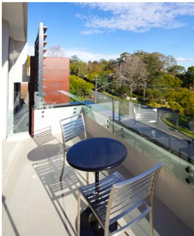
Figure 4P.5 For one and two bedroom apartments, balconies should be at least 2m deep to allow enough space for a small table
